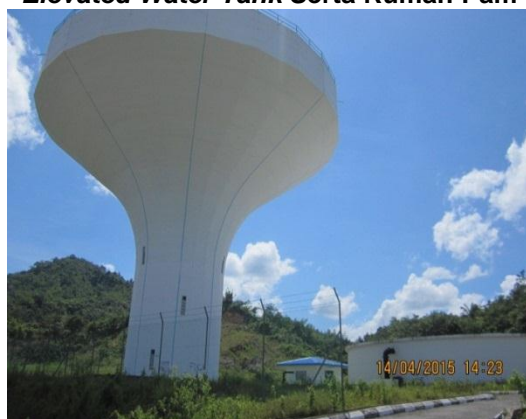
Gambar 1.3 Water Reticulation Termasuk Ground & Elevated Water Tank Serta Rumah Pam
